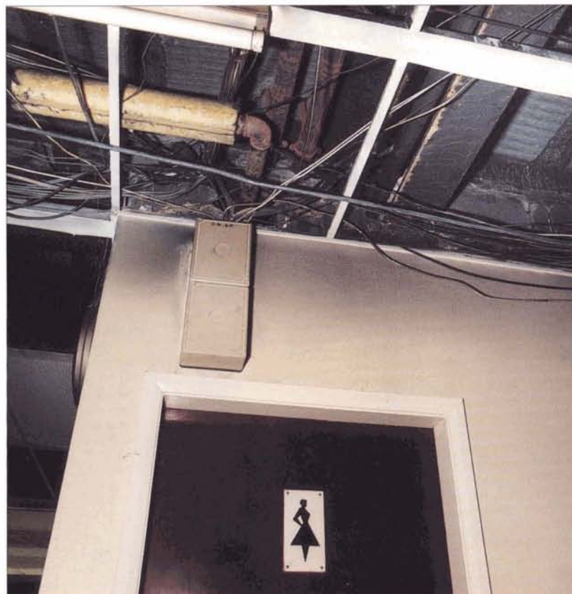
Figure 12 Photograph showing breaches in the fire-resisting enclosure around pipework and cables
