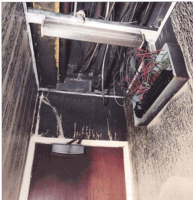
Figure 11 Photograph of smoke damage in the second floor women's toilets
